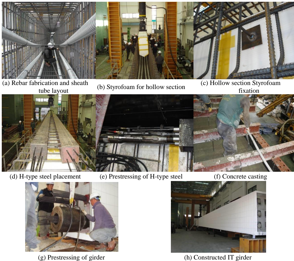
Fig. 3 IT Girder construction procedure
